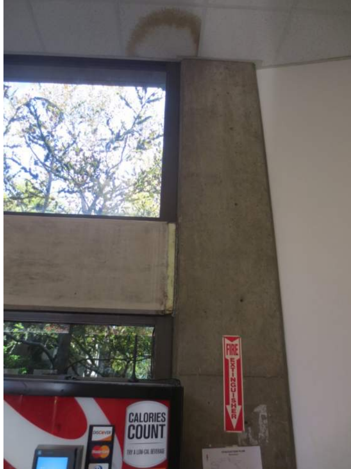
Photo 4 - Suspended Ceiling Continuous Across the Seismic Joint
