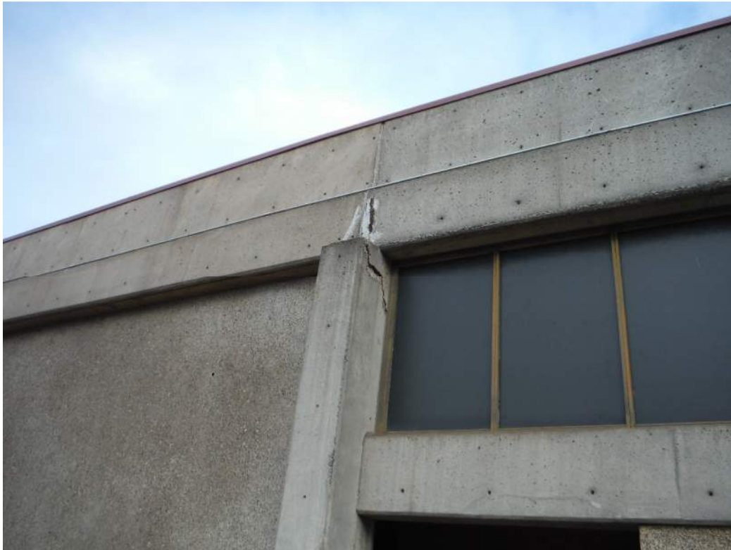
Photo 1 - Spalling of Concrete at North Entrance
