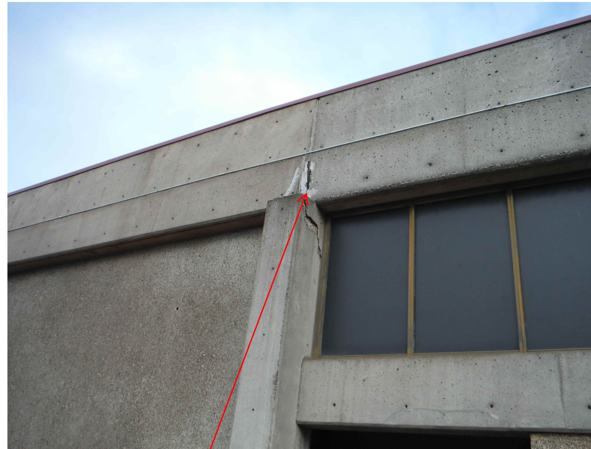
REPAIR SPALLING AT LOCATION ABOVE DOOR ON NORTH SIDE OF BUILDING.
