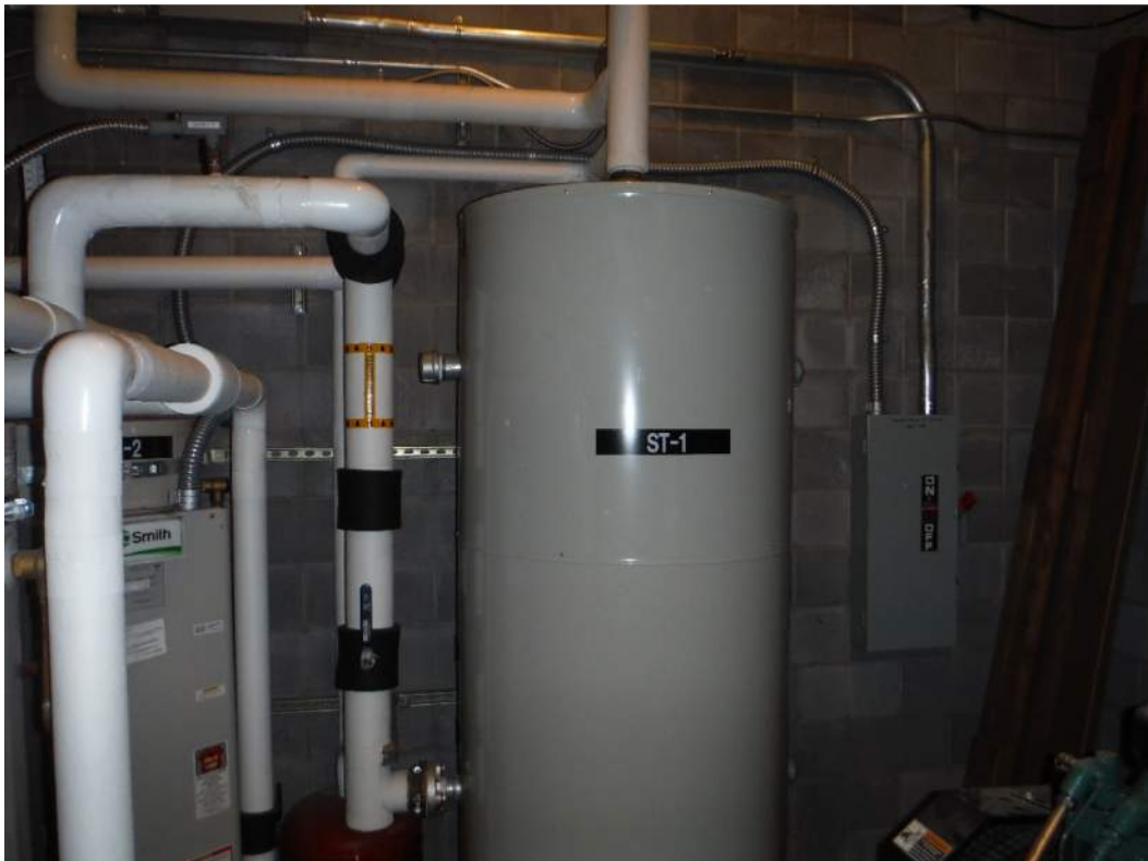
Photo 7 - Unbraced Hot Water Heater
