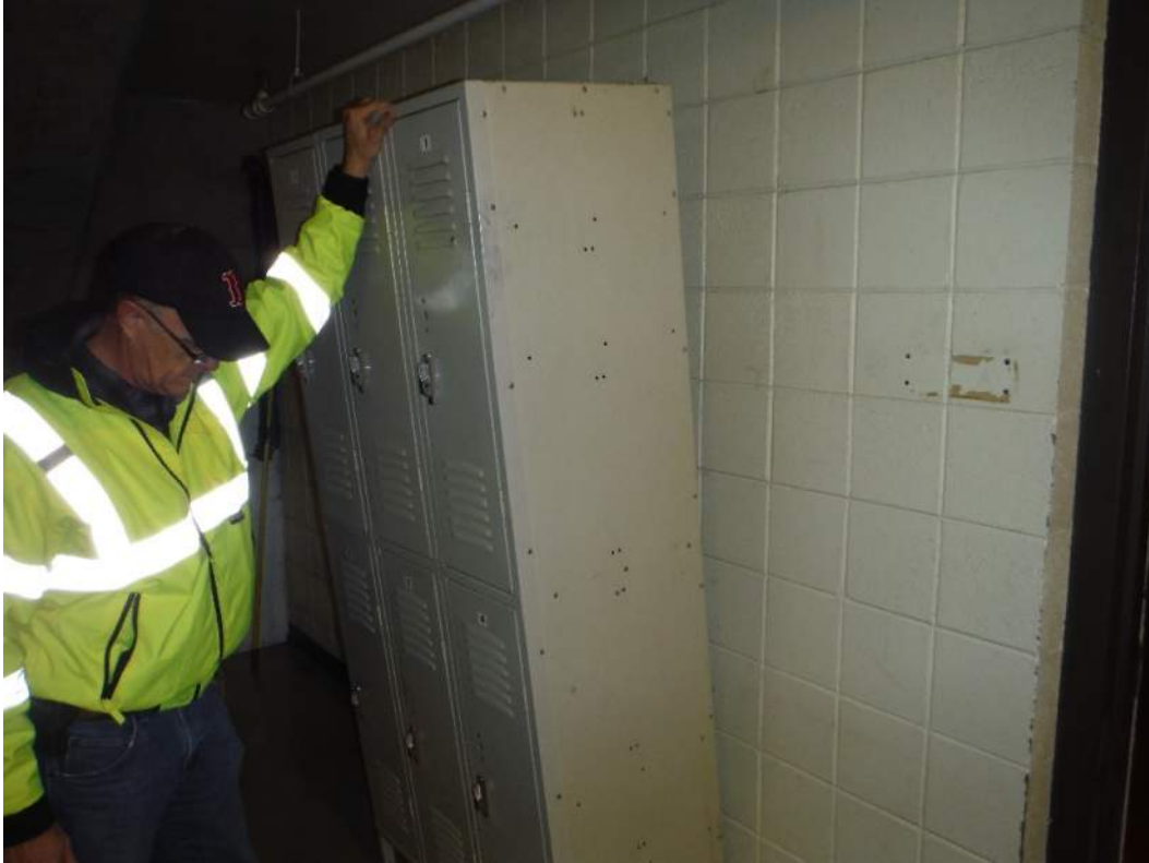
Photo 6 - Example of Unbraced Furnishings
