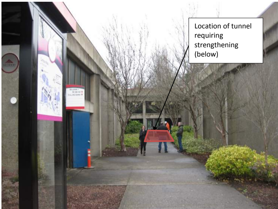
Photo 3 - Location of Tunnel Slab Requiring Strengthening
