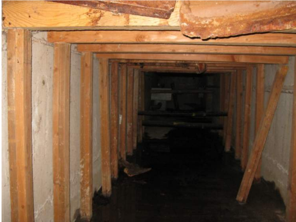
Photo 2 - Section of Tunnel Where Slab has been Repaired
